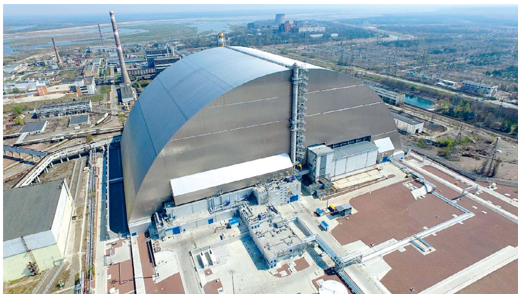
Fig. 4. New Safe Confinement
