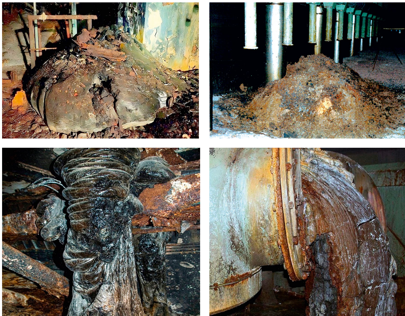
Fig. 5. Fuel-containing materials accumulations
