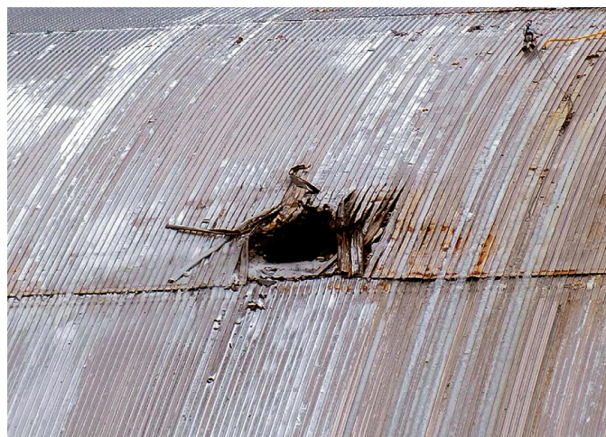
Fig. 7. Impact site of a Russian combat drone on the NSC
